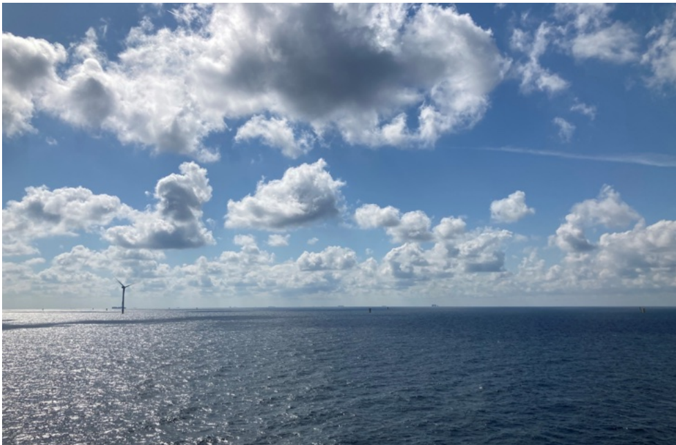
A sunny day in a North Sea offshore wind farm
